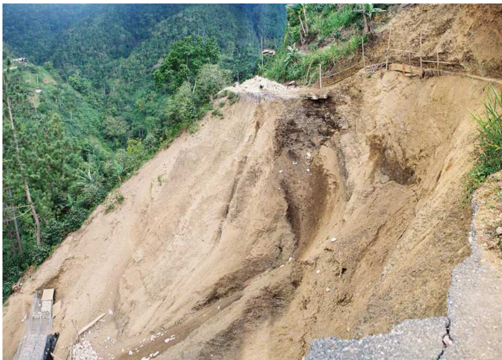
Figure 11. Landslide on the B1 road at Section in Portland Parish, Jamaica. This event severed much of the local coffee production industry from the ports used to ship the product to market. (This picture is a photo-collage and some distortion is inevitable.)
