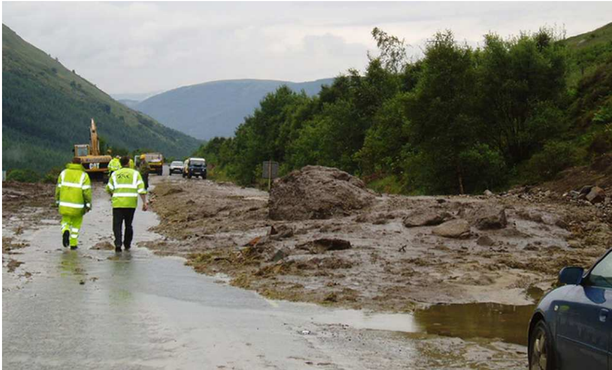
Figure 2. Debris fan containing boulders (estimated up to nine tonnes) at the A83 Cairndow event, dated 9 August 2004.
