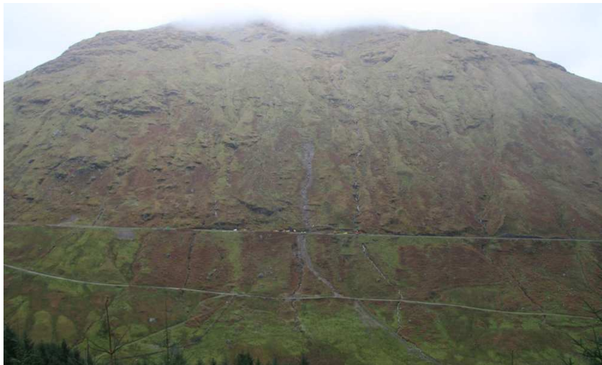
Figure 5. View of the hillside above and below the approach to the Rest and be Thankful from the east (from NGR NN 23160 06559 on the opposite side of Glen Croe). Not only can the event dated 28 October 2007 be clearly seen but evidence of numerous past events can be seen on the surrounding hillside.
